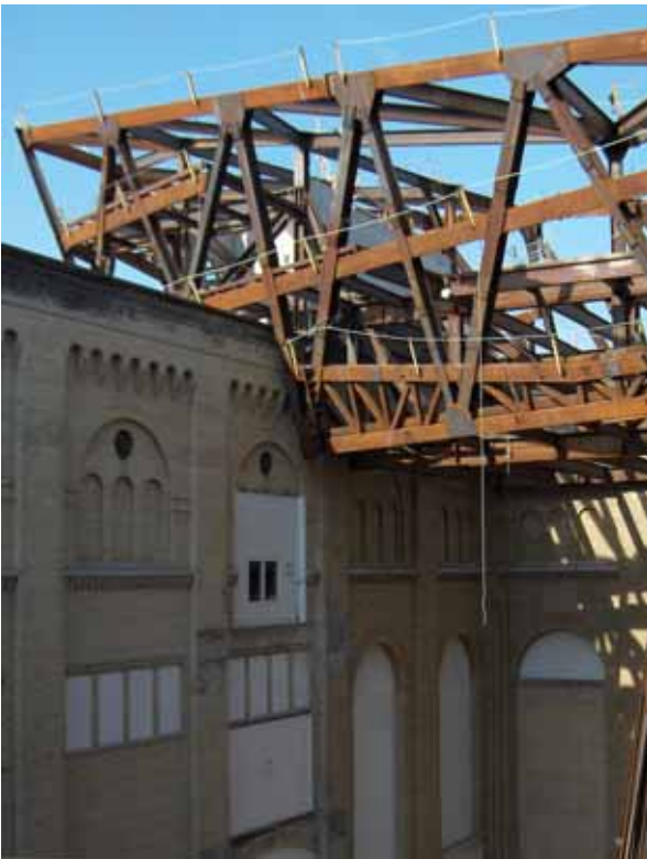
7. Crystal 5 oversailing the original building.
