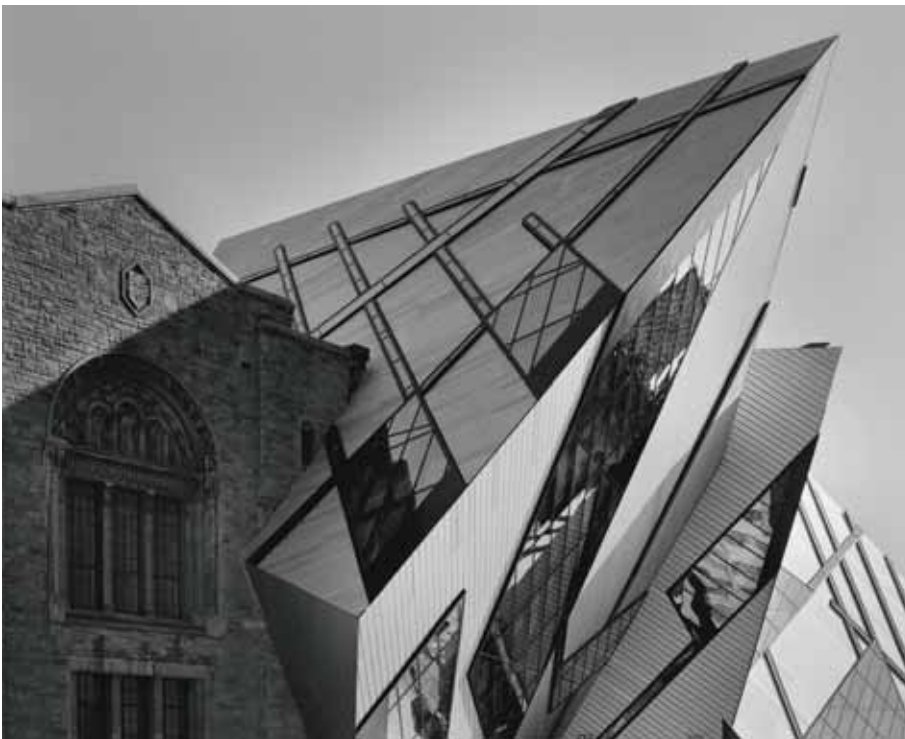
20. The completed Crystal 3 intersects spectacularly with the existing building.
