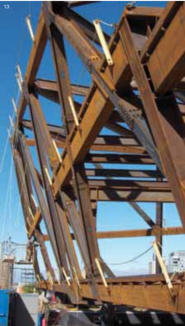
12. New frame adjacent to original building. 13. Crystal 5 spanning the original building. 14. Frame tailored to suit cladding arrangements. 15. Frame springing from "blockbuster" basement level.
