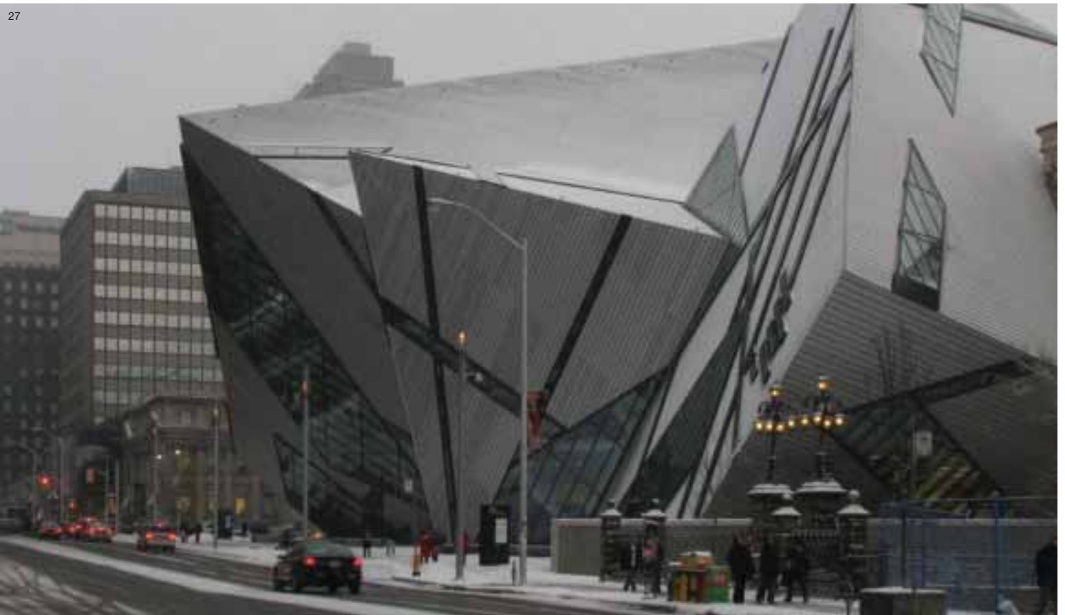
The differing natural light of the seasons (Fig 26 summer; Fig 27 winter) creates a range of visual effects on the Crystal exterior, as does projected illumination during the hours after dusk (Fig 28). Toronto's other icon, the CN Tower - until recently the world's tallest freestanding structure - can be seen top right.
