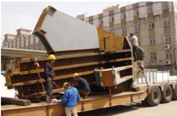
9. Delivery of column baseplate, April 2006.
