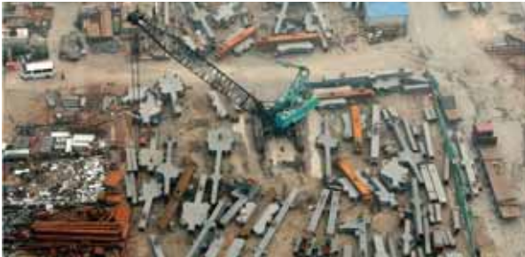
13. Prefabricated elements stored on site.
