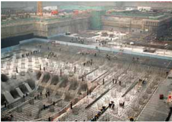
8. Preparation of foundation raft.
