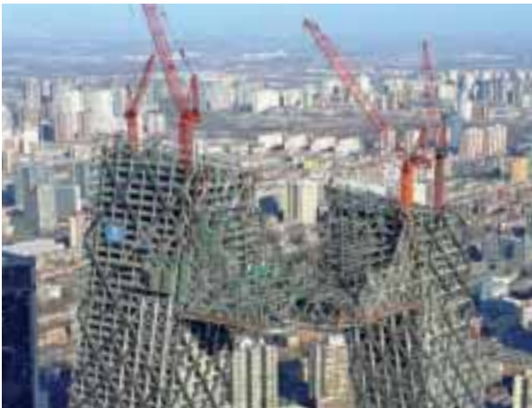
23. Installation of first connection element.
