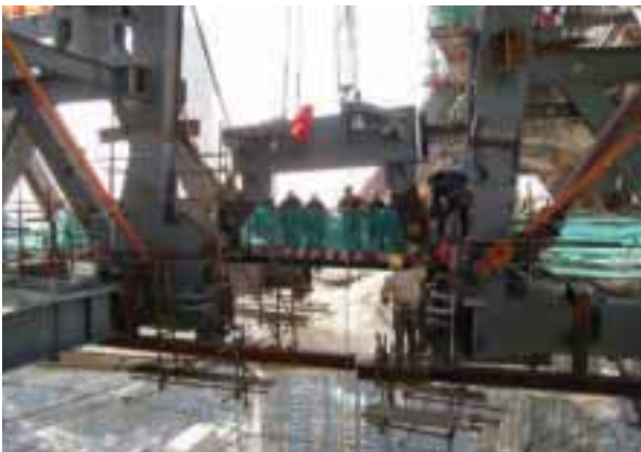
23. Installation of first connection element.
