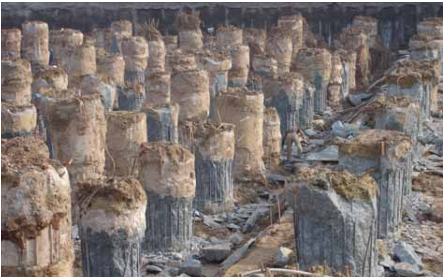
7. Cutting down piles by hand.
